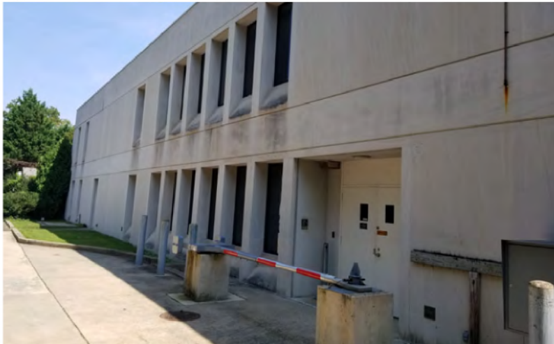
Fig. 1.6.5 - Existing public alley facade
