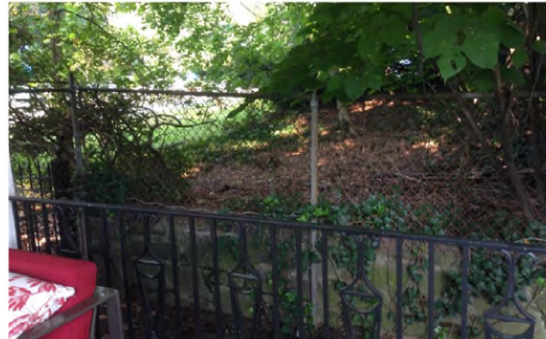
Fig. 1.6.4 - Existing perimeter fence
