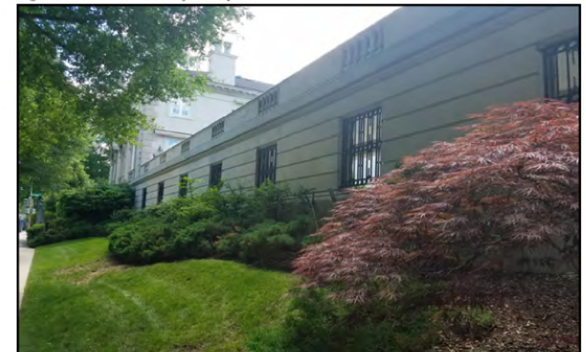
Fig. A-1.1.3 - Existing Garden wall and Residence
