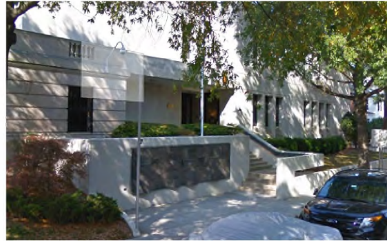
Fig. 1.6.2 - Existing entry along 34th Street
