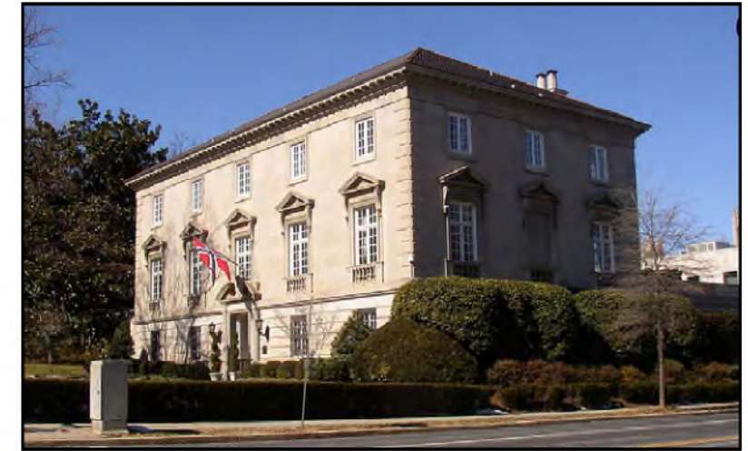
Fig. A-1.1.1 - Existing Ambassador's Residence
