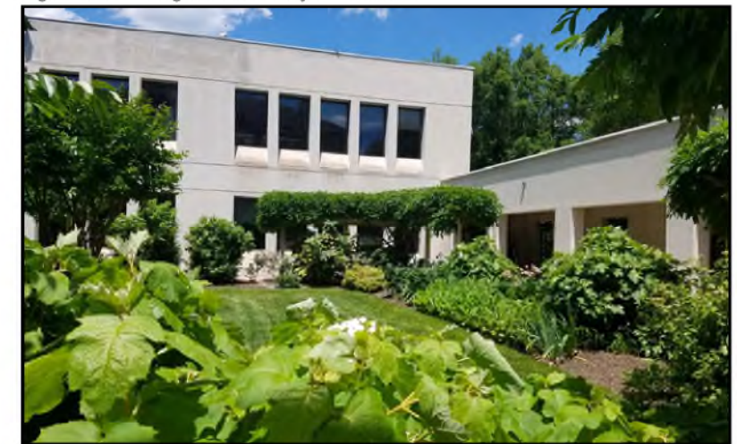
Fig. A-1.3.2 - Existing Garden Facade of Chancery
